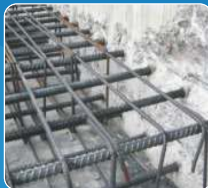
WALL TO SLAB CONNECTION
